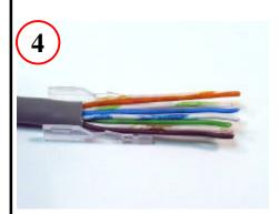
Lay wires into approx. positions in Load Bar
